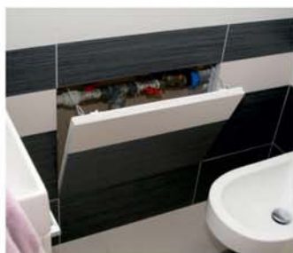
Example of installation: Consignment without tiles.
